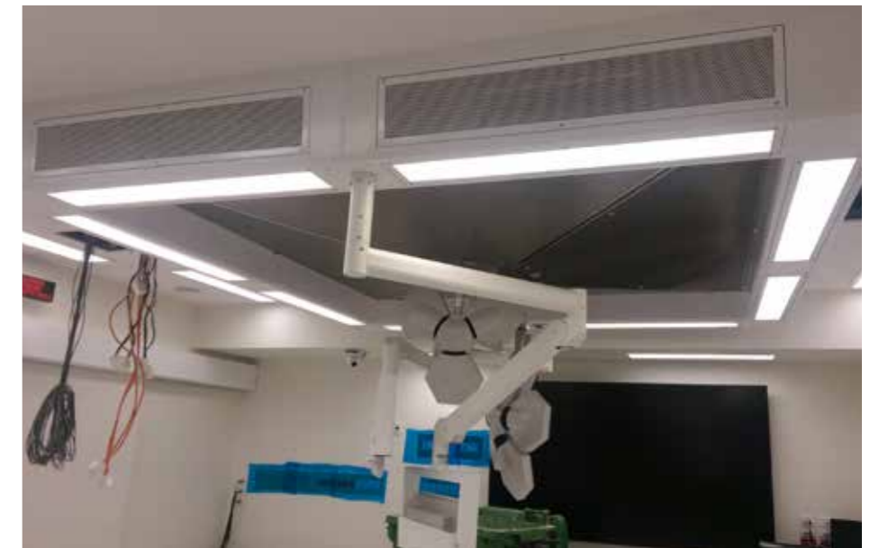
FOCUS 3000 bulkhead style installation, shown with integrated fluorescent perimeter lighting and return air facilities.
