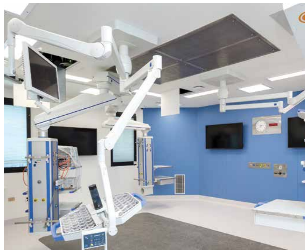
Hybrid FOCUS installation, shown with joined terminal HEPA modules
